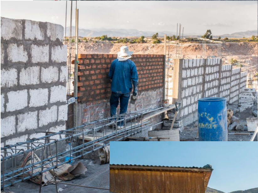
Using standard bricks to build the wall over the cistern.
