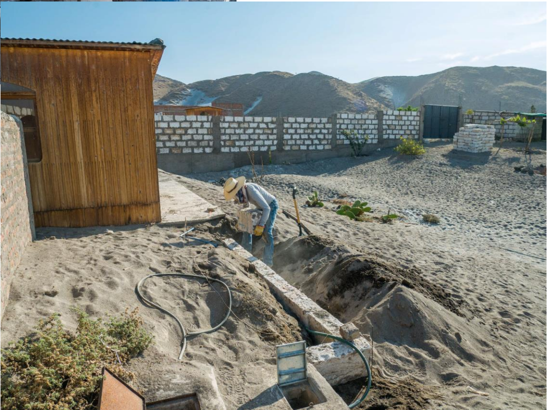
Using standard bricks to build the wall over the cistern.
