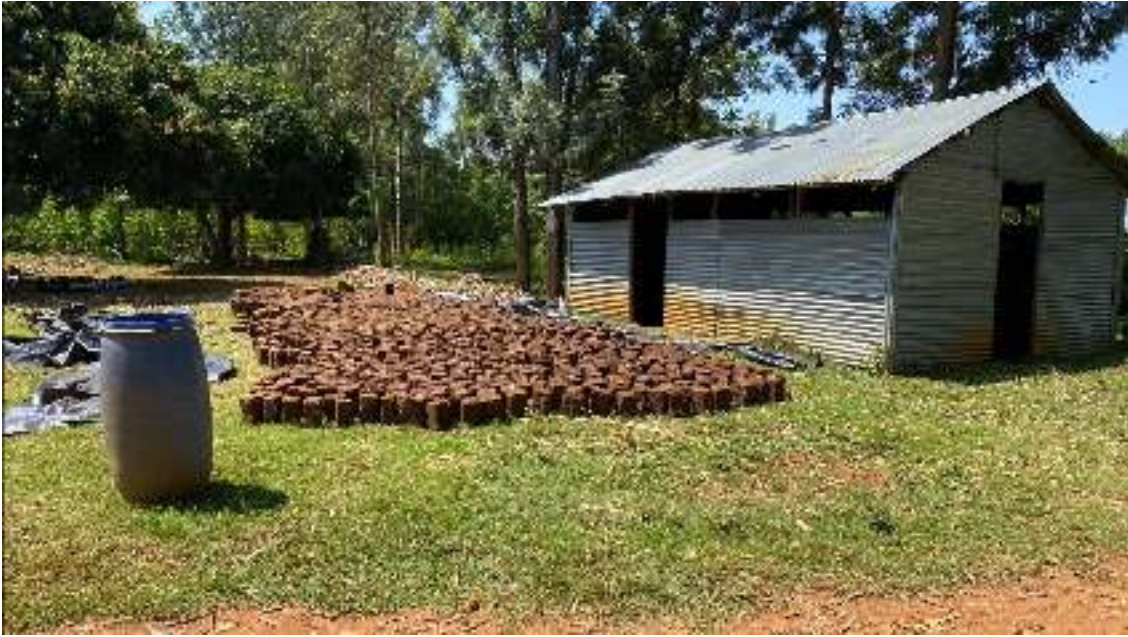
Pastor Mike is taking this time during Covid 19 to make bricks for replacing the old church building.
