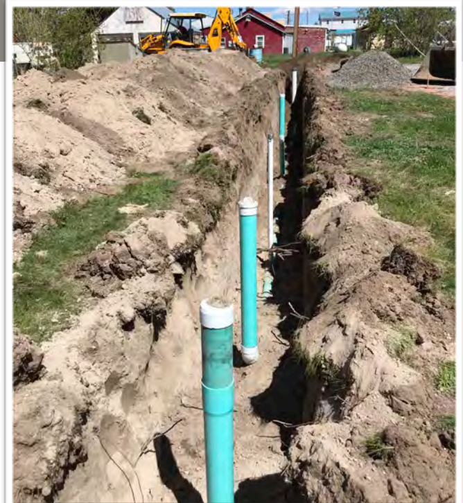
Sewer line rough-in on our property
